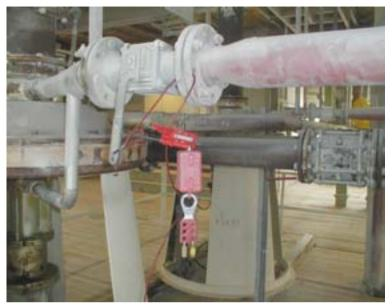
Lockout on a pipe to prevent unintentional release of hot stem. The master lock in the red box blocks the clip. The master lock cannot be removed before the two workers have removed their personal keys
