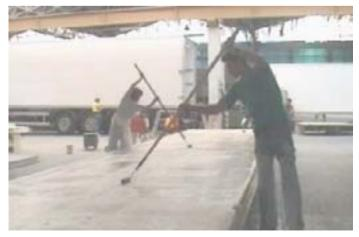
Before: resin spreading with rollers
