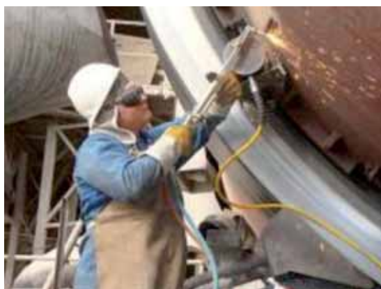
Maintenance work involving welding
