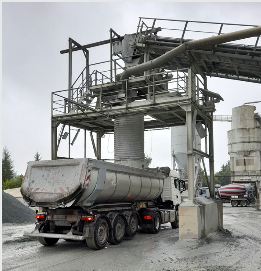
Figure 15-5: Height-adjustable truck-loading spout with dustproof skirt
