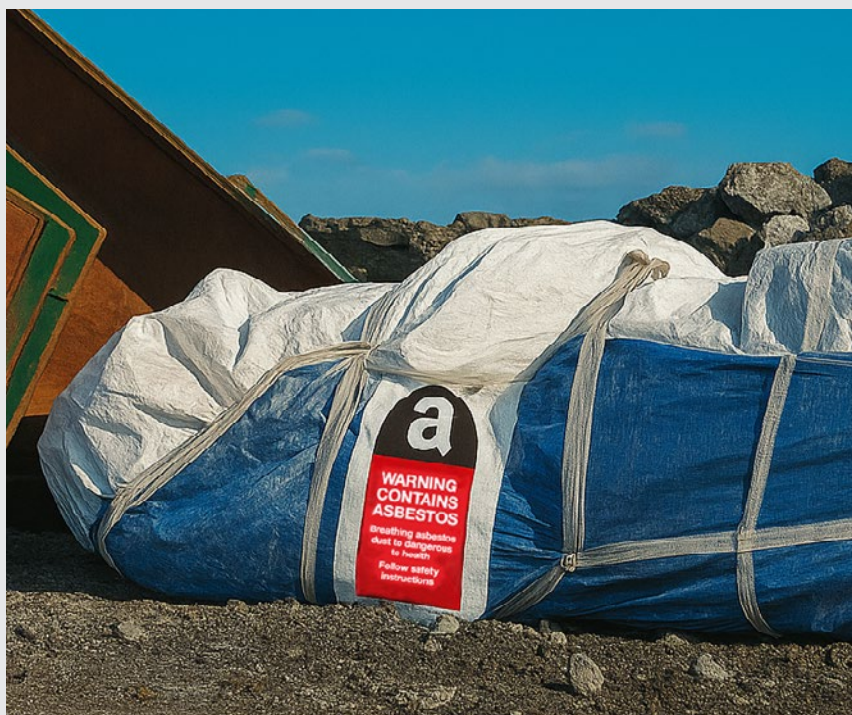
Figure 12-3: WCA disposed in sealed bags
