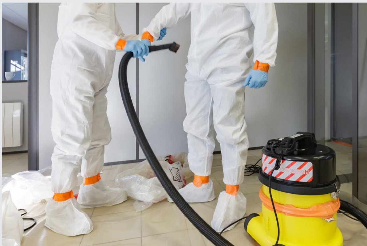
Figure 8-6: Example of cleaning using a vacuum cleaner
