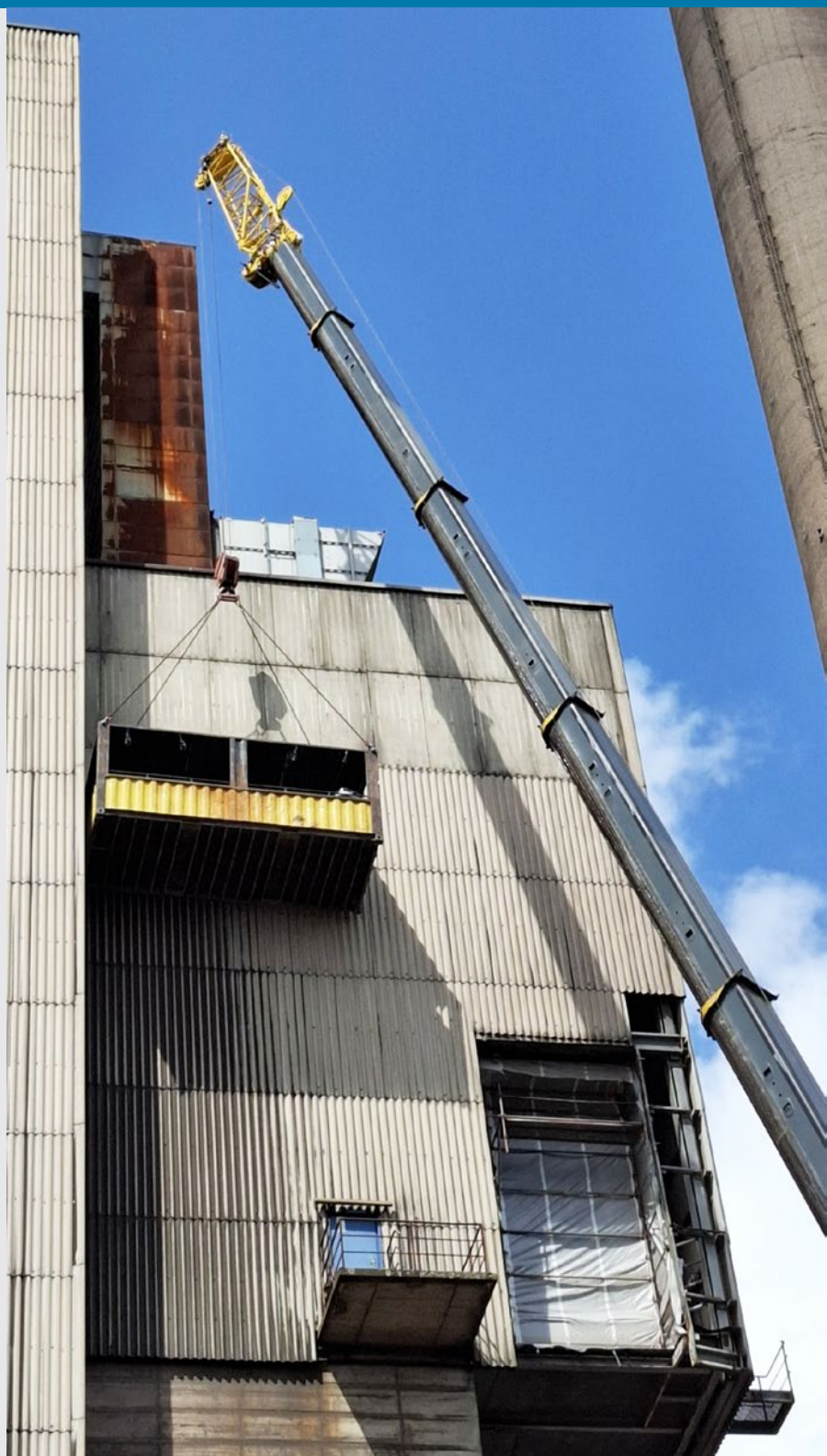
Figure 4-2: Example of the risk of working at heights during the removal of asbestos plates during the demolition of a power plant in Germany
