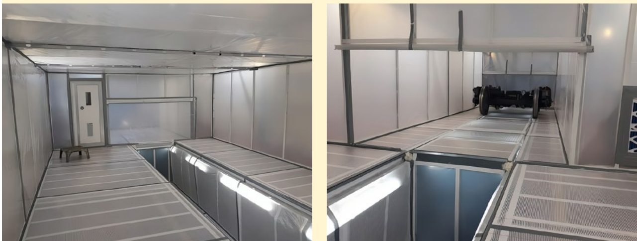
Figure 14-4: Large containment unit with a pit for bogies
