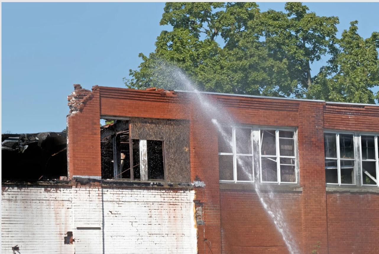
Figure 8-1: Example of wetting a building containing asbestos
