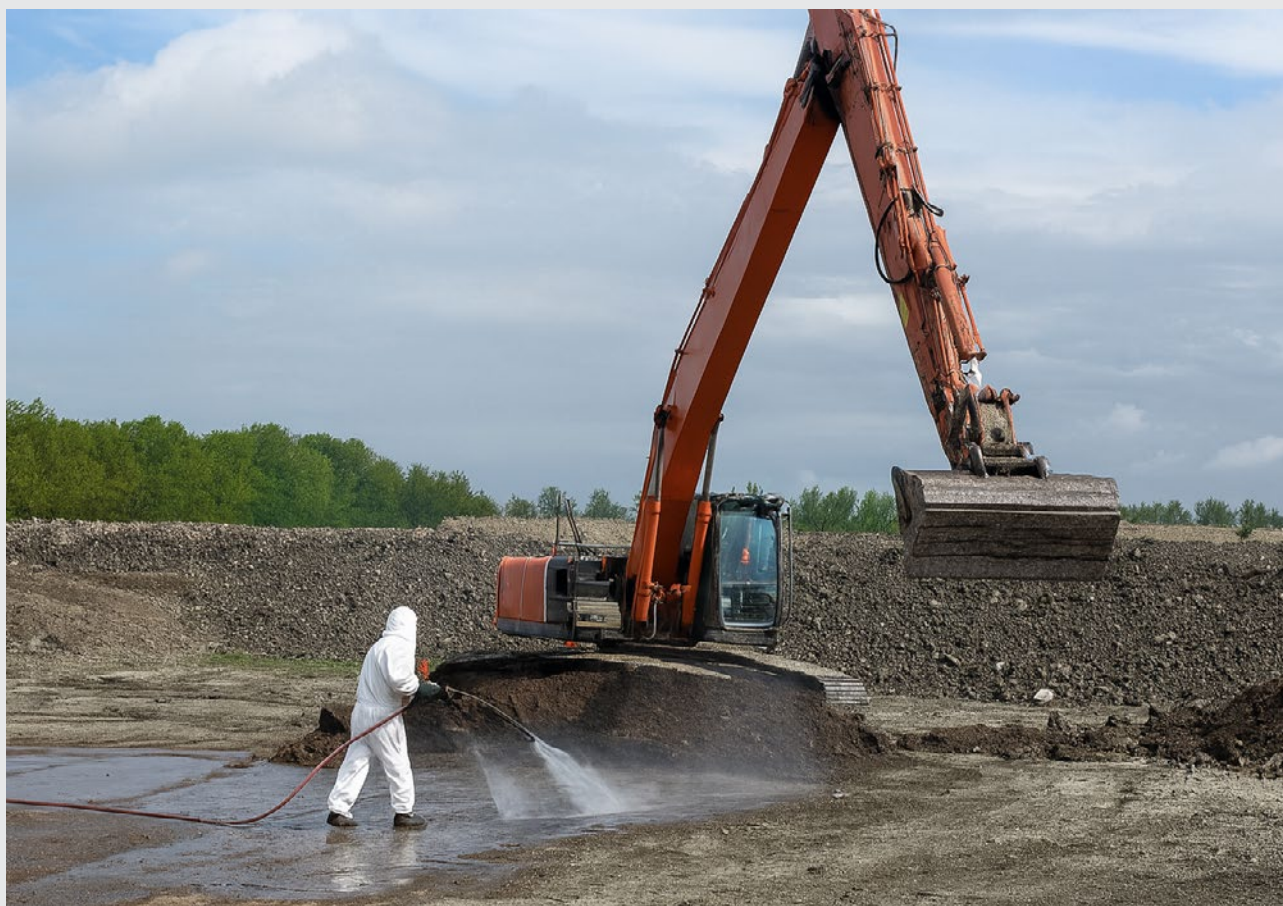
Figure 12-2: Wetting of WCA to prevent dust
