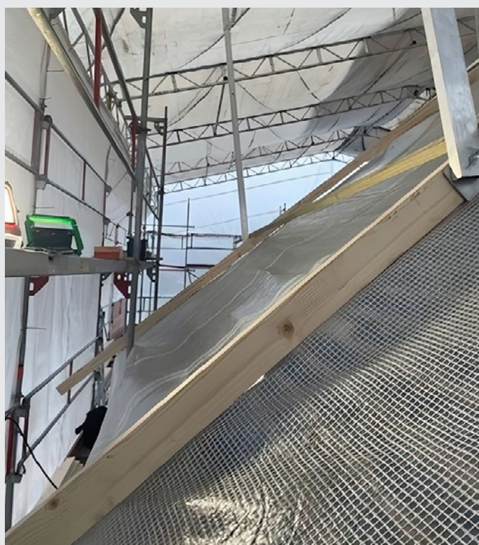
Figure 13-4: Suspension system inside an asbestos tent
