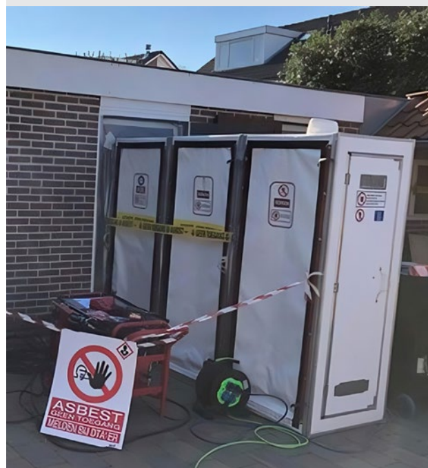
Figure 8-5: Example of a decontamination unit set-up
