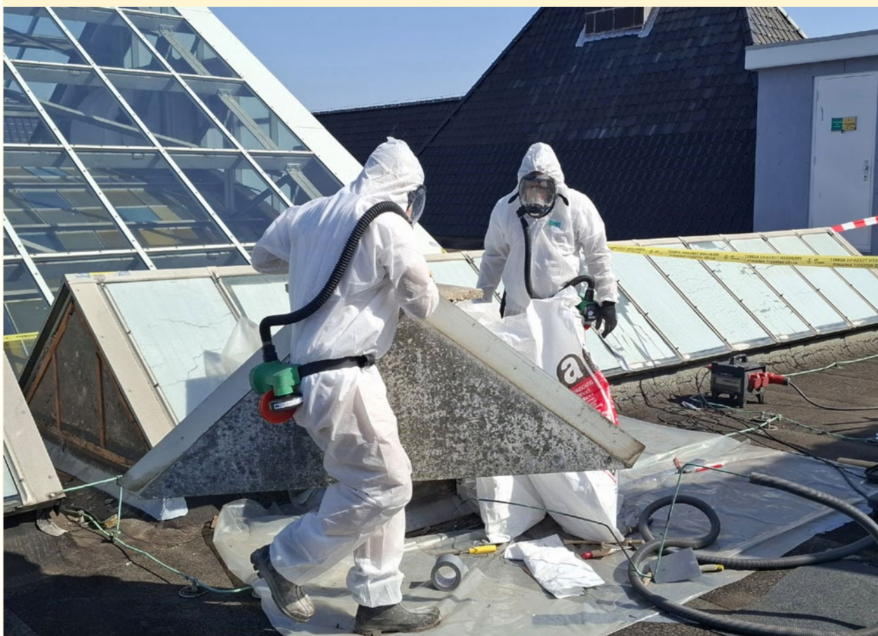
Figure 4-4: Workers removing asbestos plates on the roof
