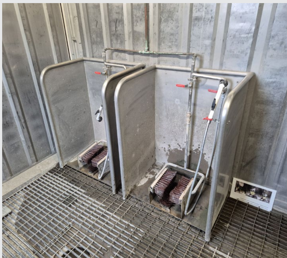
Figure 15-3: Footwear washing facilities inside a decontamination chamber
